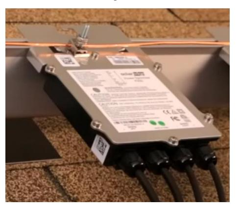
Optimizers increase energy output from PV systems by constantly tracking the maximum power point (MPPT) of each module individually.
