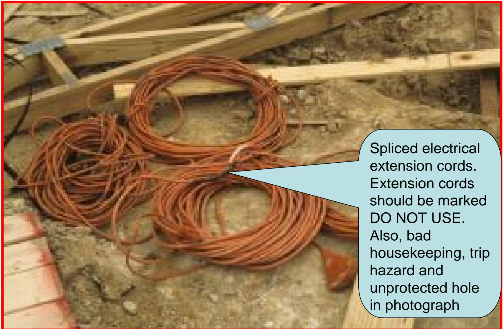
Spliced electrical extension cords. Extension cords should be marked **DO NOT USE**. Also, bad housekeeping, trip hazard and unprotected hole in photograph
