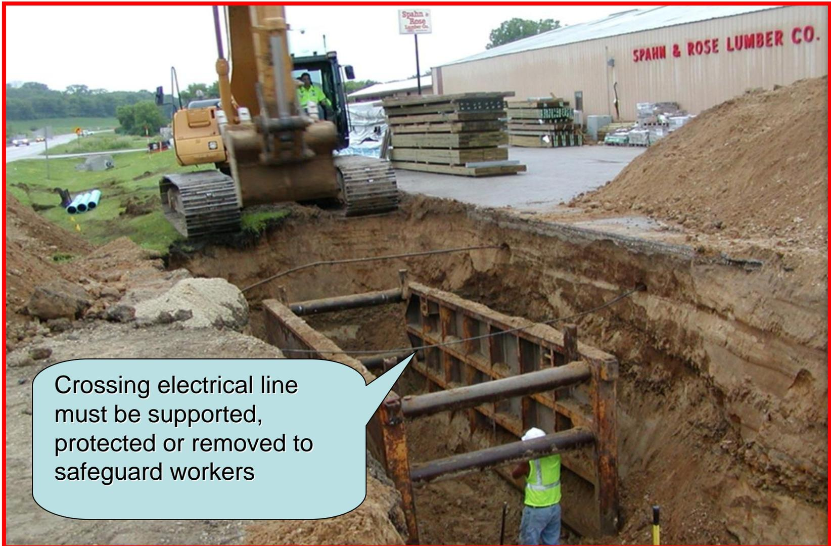
Crossing electrical line must be supported, protected or removed to safeguard workers
