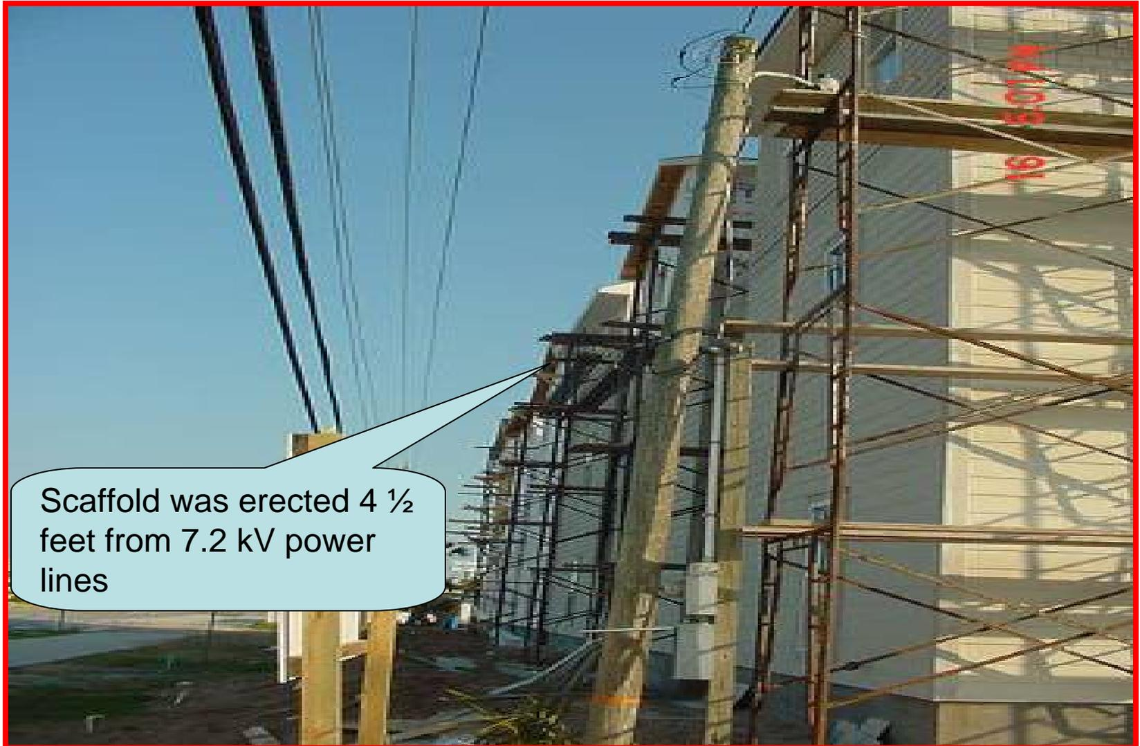
Scaffold was erected 4 ½ feet from 7.2 kV power lines
