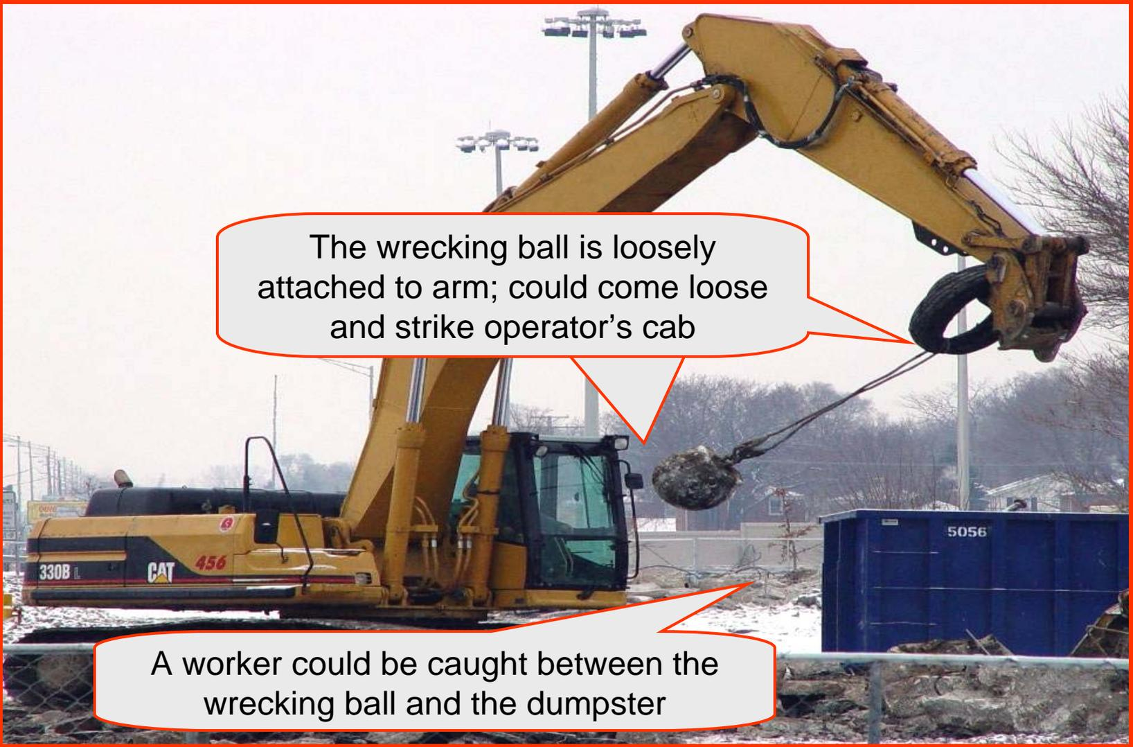
The wrecking ball is loosely attached to arm; could come loose and strike operator's cab
